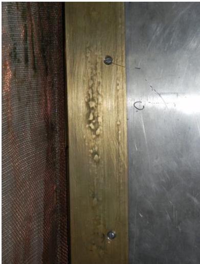
Gap between two screw at least two inches is required.
