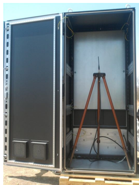
Fig.2 Receiver antenna inside rack
